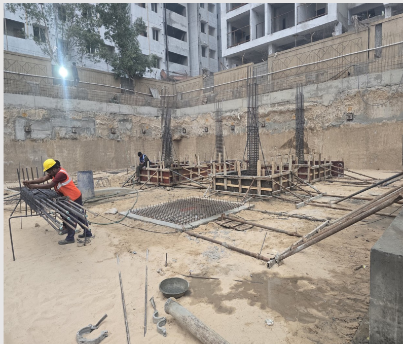
Building foundation and column footing casting work in progress.
