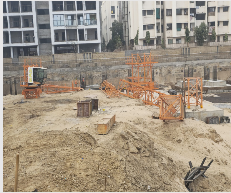
Tower crane installation.
