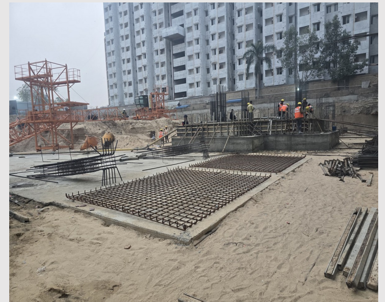
↓ Building foundation being cast.
