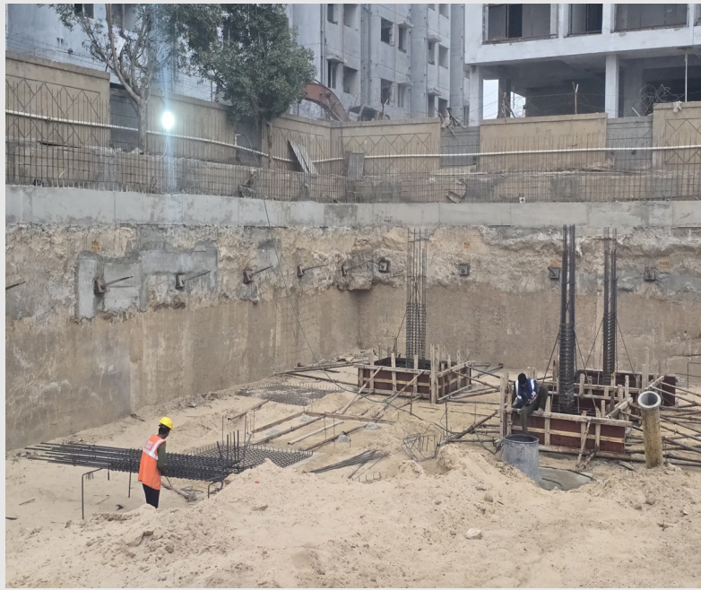
← Diaphragm wall that is cast around the basement.
